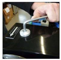
Fig. 1 - Remove top mounting screws
